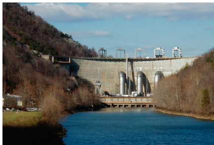
Looking upstream at Smith Mountain Dam
